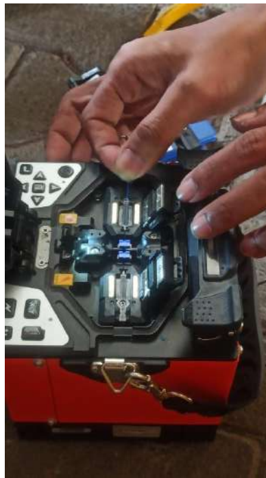
Lampiran 5. 5 Splicing fiber optic
