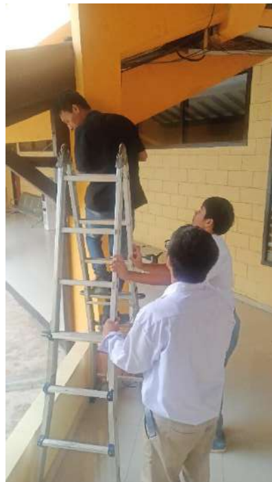
Lampiran 5. 10 Menarik kabel fiber optic
